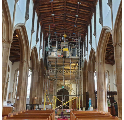
Strengthened scaffolding in place
