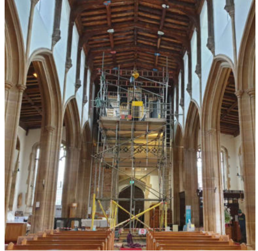
Strengthened scaffolding in place
