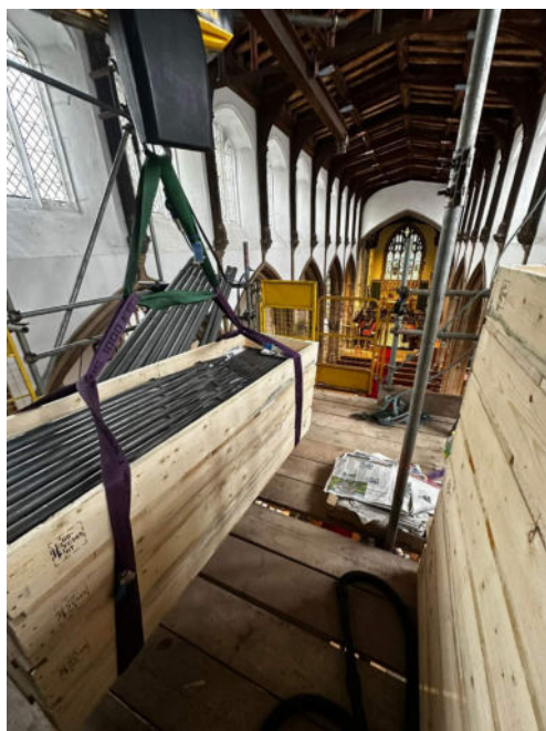
Pipes carefully packed for re-use.
