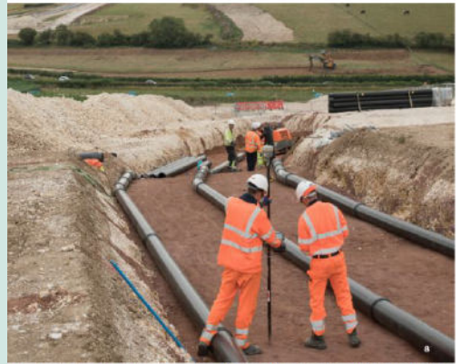
NG - Construction best practice for underground cable installation
