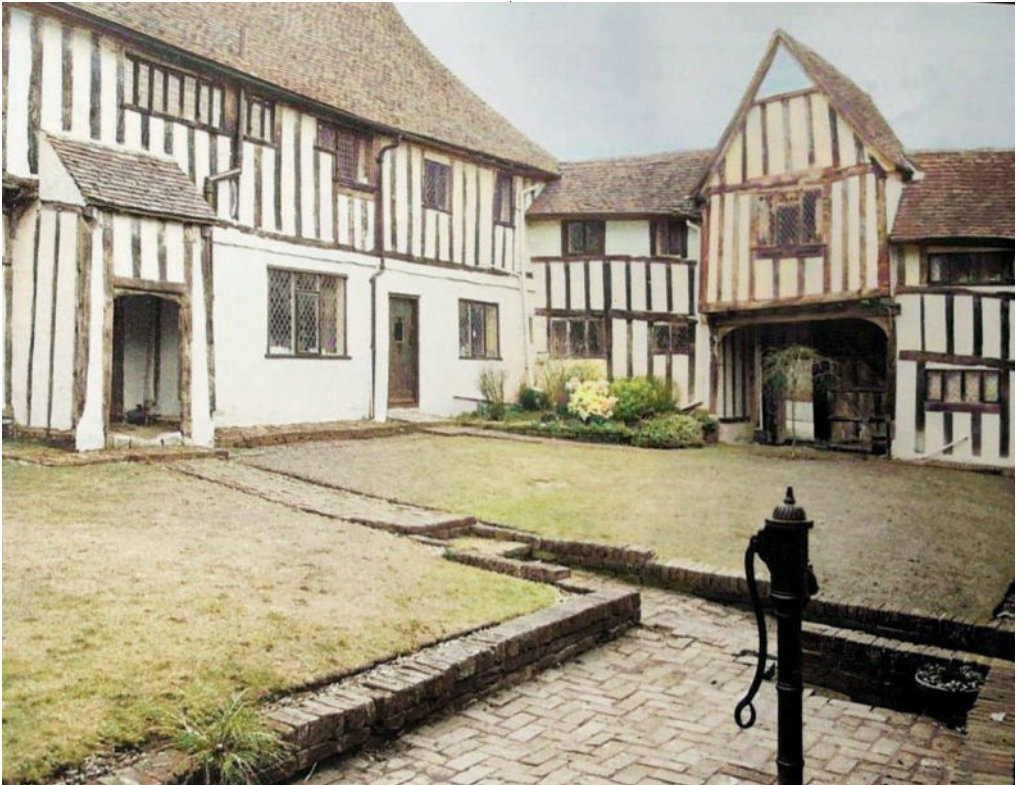
Courtyard after restoration.
