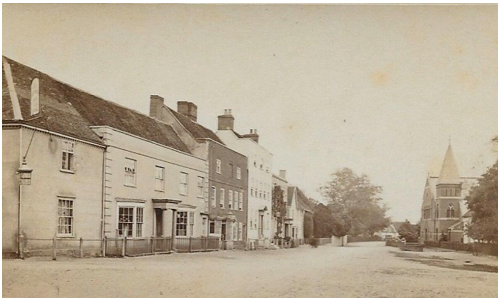
A late 19th-century view of Royal Square showing the Marlborough Head Inn on the left with its massive roof shared with Church (now Loom) House next door. Note the bay windows on the house, which were replaced by shop windows in the 1890s but reinstated in the mid twentieth century.
