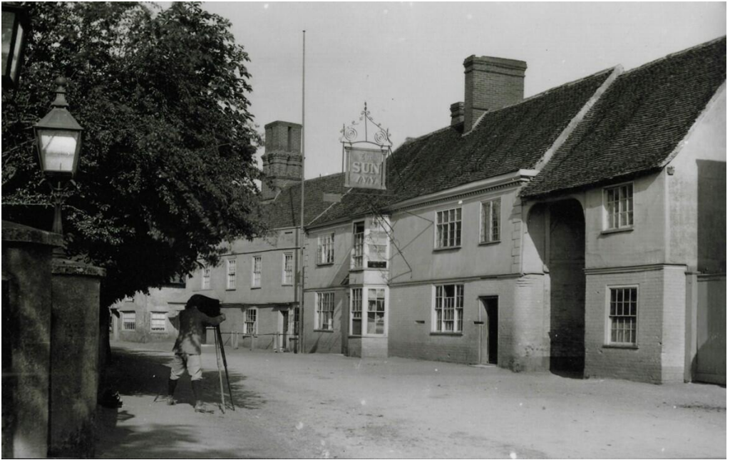
A photographer outside the Sun Inn in the 1890s. Note the squints on either side of the window to the left of the arch, which allowed grooms waiting in the bar to look out for approaching coaches.
