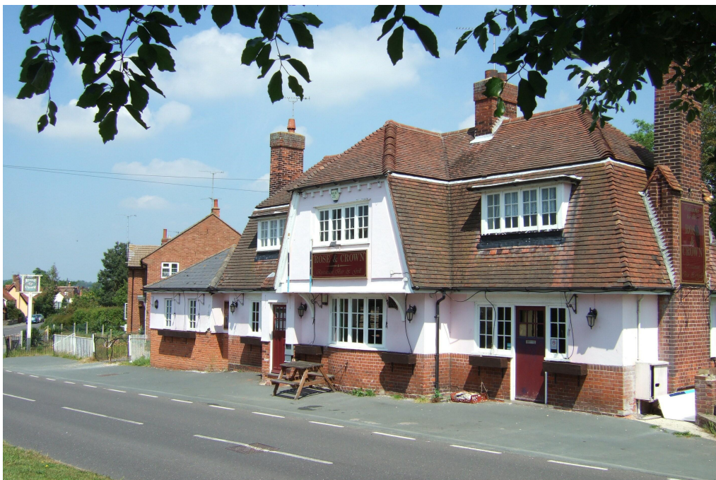
The Rose and Crown as rebuilt in the 1930s. It closed down in 2009 and was demolished.
