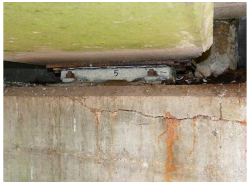
One of the temporary jacking frames installed on the South abutment ready to be jacked-up to lift the bridge deck off the bearings.
