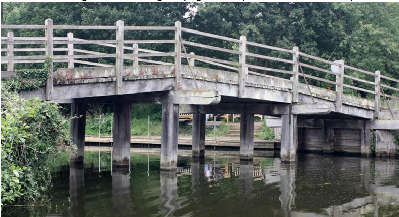
Flatford bridge, a replica of the original bridge constructed in Burmese wood in 1951, illustrating the traditional construction of bridges along the Stour
