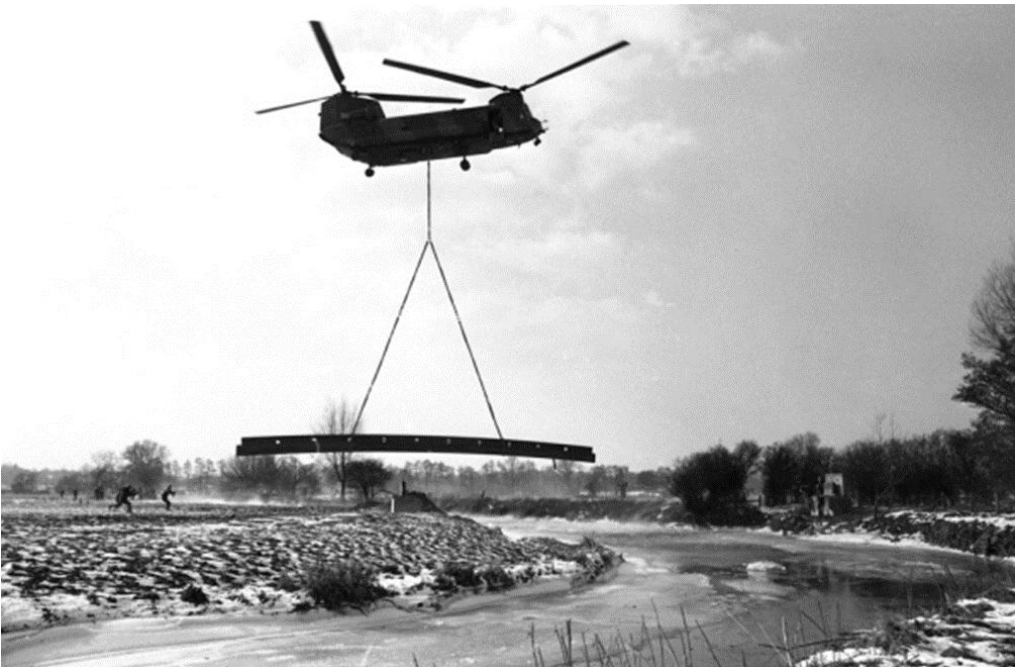
Fen Bridge in the early twentieth century. Lifting the new Fen Bridge into place, February 1985
