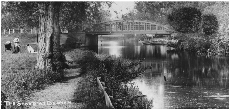
Dedham's iron bridge installed in 1900.
