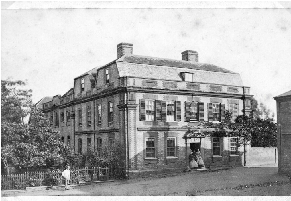
Members of the Lermitt family on the doorstep of the Grammar School in the 1860s. Note (far right) the corner of the recently-built Duchy House
